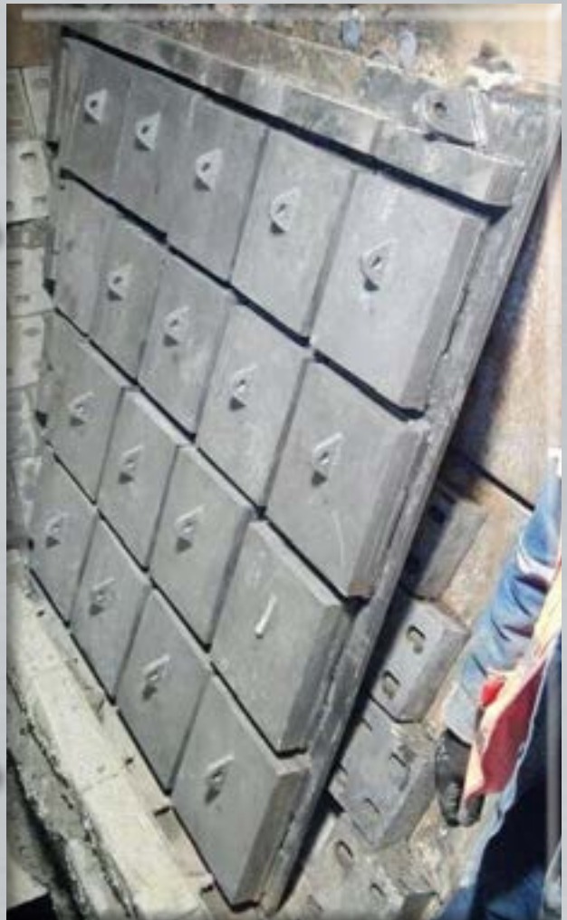
Lock Liners installed in position using a pre-assembled backing plate
